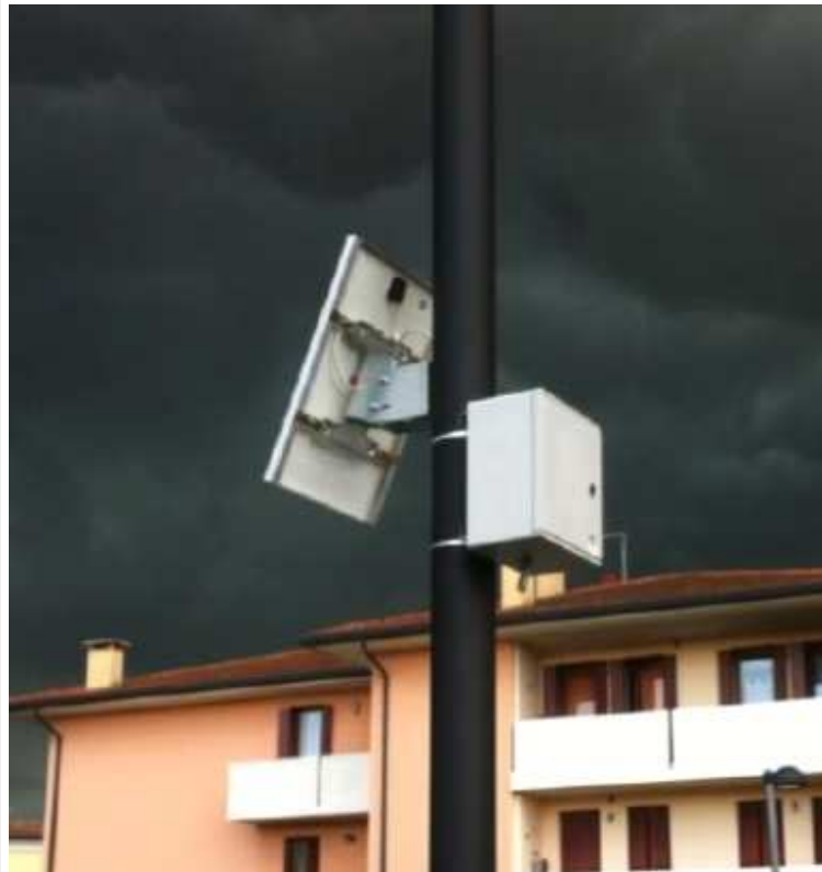
Fig. 3.2. Access Point installation
