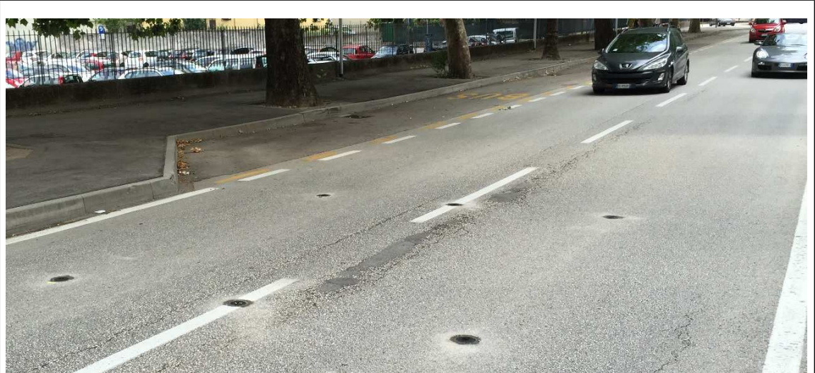
Fig. 5.2. TDM WI sensors detecting vehicles approaching an intersection
