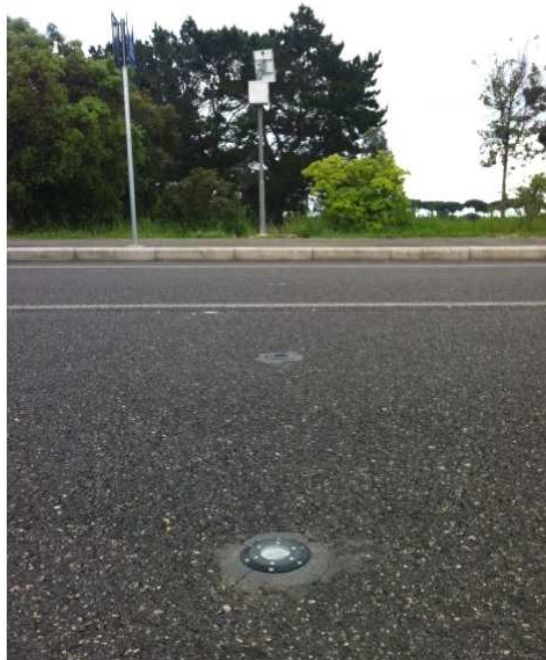
Fig. 5.5. TDM WI sensors detecting vehicles approaching an intersection & System Hub
