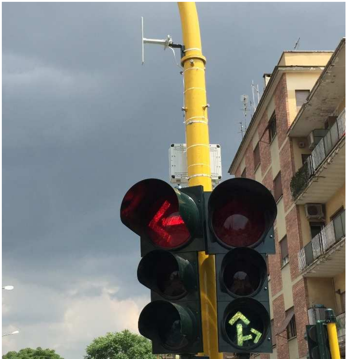
Fig. 5.6. TDM System Hub & Access Point
