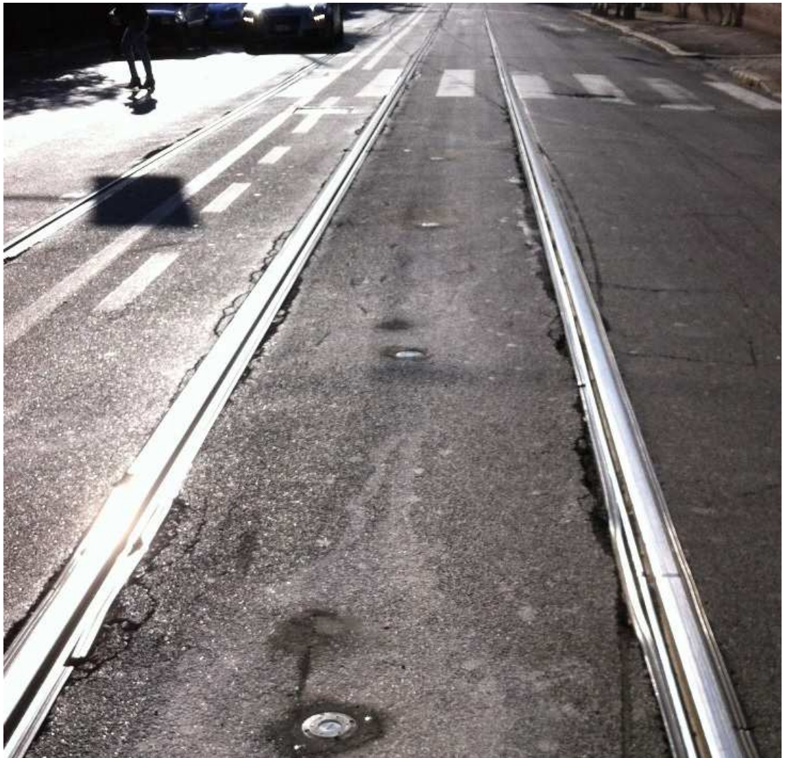
Fig. 5.1. TDM WI sensors for a light railroad control
