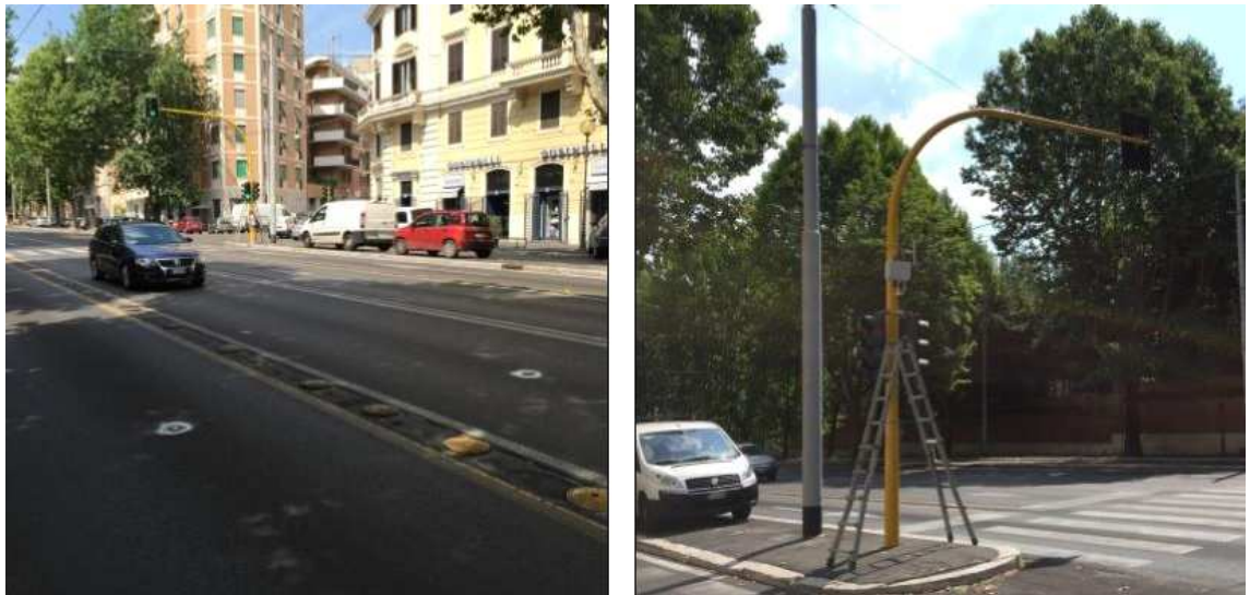
Fig. 5.4. TDM WI sensors detecting vehicles approaching an intersection & System Hub
